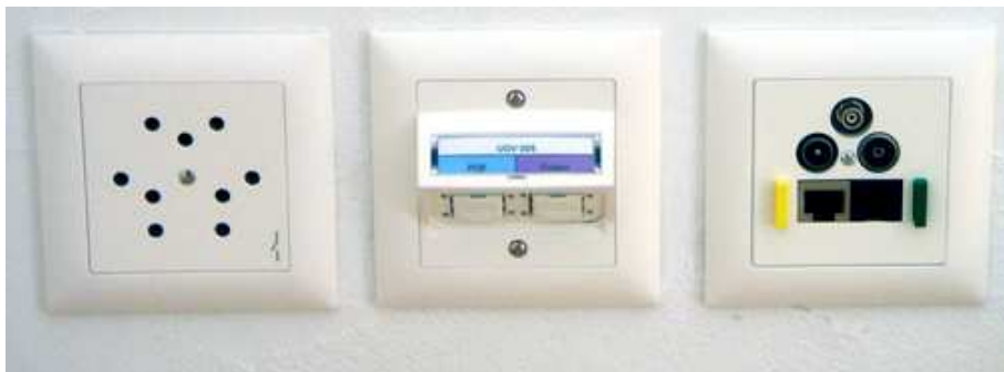
Fig. 4.2.3: Example of a group of sockets with (from left) Power, TO, MATO. Photo: R&M
