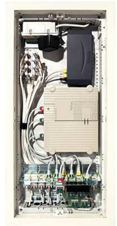
Fig. 3.1.1: Communication distributor – interface between the house entry point and the home network. Photo: R&M
